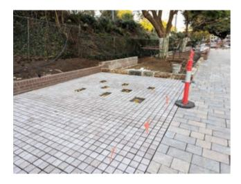
The recent transformation of Artarmon Village Green has been a highlight with works including the reinstallation of the sandstone kerb, new concrete gutter, paving, street furniture, feature walls, and shared path completed. Fresh topsoil has been prepared for mass planting which will be commencing soon.
