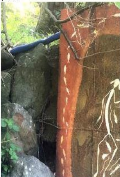
Blue pipe leading from houses to drain and FR Creek next to shared path
