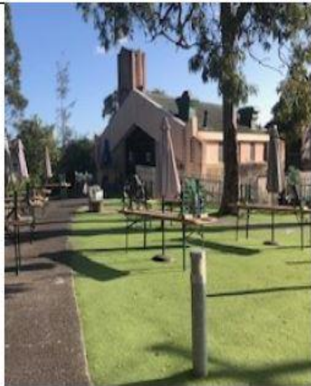
Unsightly rubble, weeds, fence at back of incinerator (see over page)
