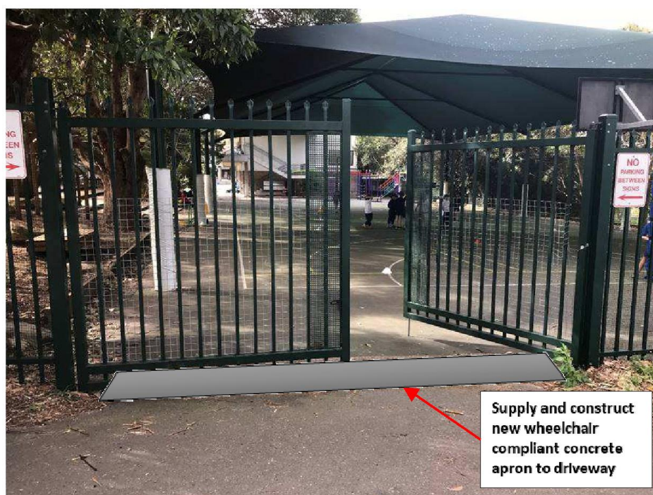
Figure 18: Double gates at Roche Lane – New concrete apron
